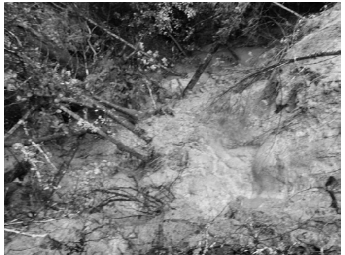
A 2006 landslide on the Cornell property caused an estimated 10,000 cubic feet of sediment to enter the Mark West Creek.
